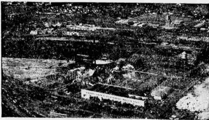
PLYWOOD PLANT AT EUGENE
