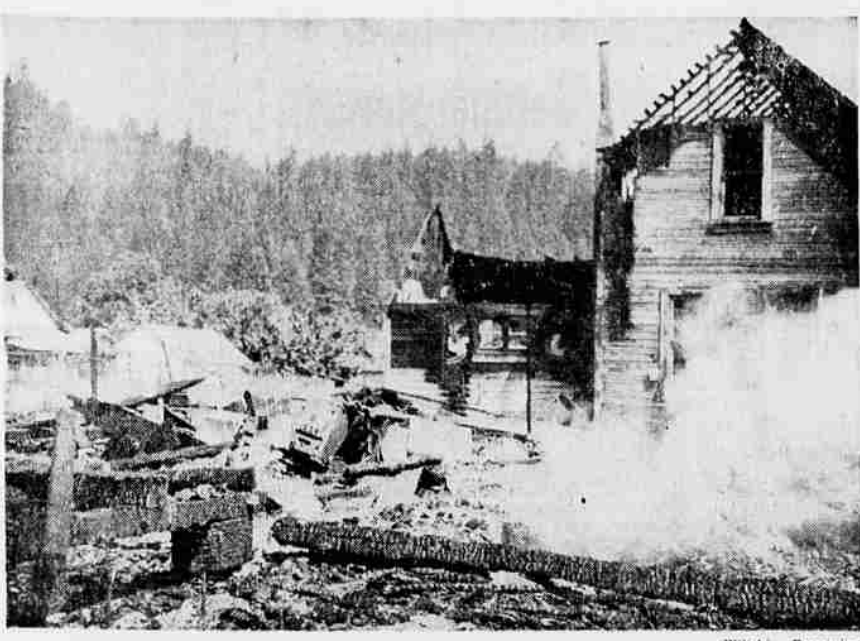
HERE ARE THE SMOULDERING ruins of the Marcola Methodist Church and parsonage, snapped Monday morning by the pastor, the Rev. Stewart Place. Neighbors of the town fought the fire all night. The standing portion of the ruin is the parsonage; the church formerly stood in the immediate foreground. Services will be held in the Victory Theater; Methodist churches are asked to donate a few Methodist hymnals, and some Sunday school hymnals are also needed; chairs for the primary and junior departments, a few tables, and a piano. Other needs have been met. Practically everything, including the church's antique pulpit Bible was lost in the fire.
