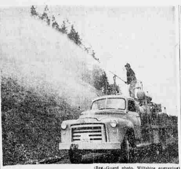
A GRASS GUN goes to work on the new Eugene-Goshen cutoff. Rudy Seigmund, State Highway Dept. grounds man, demonstrates the high-powered seeder on the banks of a cut just north of the Goshen underpass. The machine is especially useful in planting slopes to prevent erosion. The new limited access highway is scheduled for use this year. The grass gun sprays a mixture of seed and liquid fertilizer.
