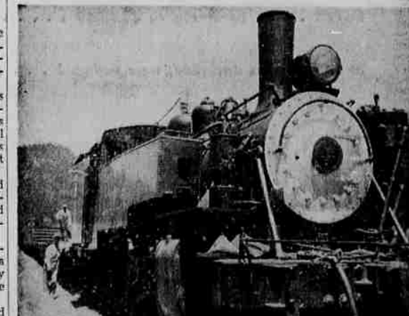
COTTAGE GROVE—"OLD NUMBER ONE SPOT," after a quarter century of faithful service up and down Row River for the Oregon Pacific & Eastern Railroad, has been retired. The old engine has never had a breakdown. In earlier days it would make three round trips a day over its 22-mile route. The 64-ton locomotive is still in good shape and will be used for "standby" service. The company's new diesel electric, "The City of Cottage Grove," will make regular runs starting Monday. (See story on page 24.)
