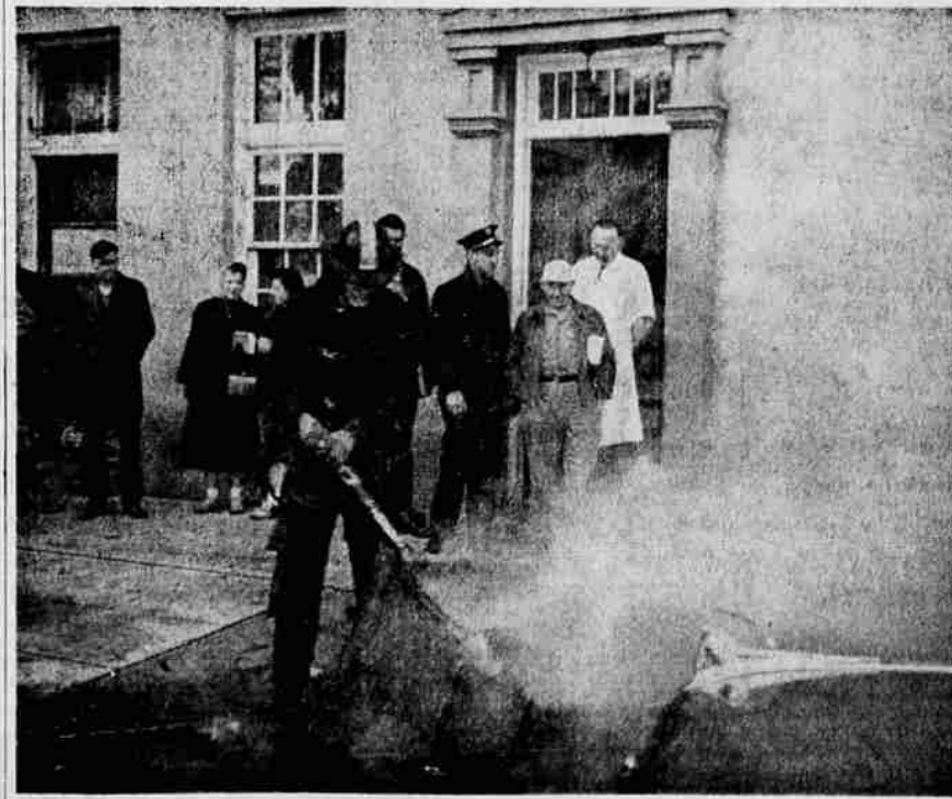
A $30,000 APARTMENT HOUSE received less than $1000 damage from fire that brought two Eugene engine companies and a truck company on the run at 3 p.m. Wednesday. The building, 583 East 13th Ave., is owned by W. C. Underwood. Fire Marshal Ed Barker attributed the fire to a cigarette on a davenport although the occupant, Robert Claypool, was not in his quarters at the time of the blaze. Glen Lyda and Charles Ferrell, who occupy apartments nearby, first noted the smoke and called in the alarm. This was the first fire loss the city has recorded since January 27. The chair was thrown from second-floor apartment to fireman on street who doused the flame.
