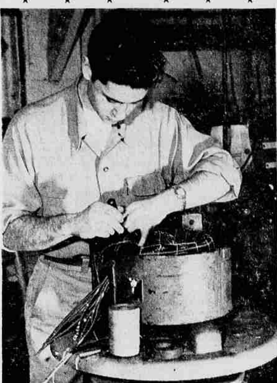
(Vocational School photo, Wiltshire engraving) THE FINAL STEP IN REPAIRING an electric motor, ty-ing in the windings, is only one phase of study in the electrical repair department at Eugene Vocational School. EVS will hold open house Thursday from 7 to 10 p.m. and Friday, 3 to 5 p.m., when displays and demonstrations of the departments will be held. Here, Ron Peppercorn is tying in the windings of a rewound electric motor.
