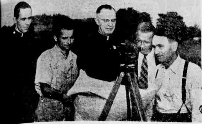
Here is a proud and happy moment for Father Francis P. Leipzig, long-time head of St. Mary's Catholic Church, as builders begin actually moving dirt for construction of the new Catholic High School, fronting on Eighteenth Avenue near Jefferson Street, just south of the fairgrounds and the municipal swimming pool. Left to right, Father J. J. Linehan, assistant pastor; S. Stien, superintendent for construction of Stien Bros., contractors; Father Leipzig; Graham Plater, architect; Roy Stien, contractor. (Register-Guard staff photo, Wilshire engraving.)
