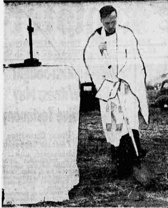
REV. STERLING SIMONSON breaks ground for the first unit of the Springfield Lutheran parish house and church project at Fourteenth and J Streets. A public block structure is now being built at a cost of about $20,000 on the 405 by 111-foot site.
