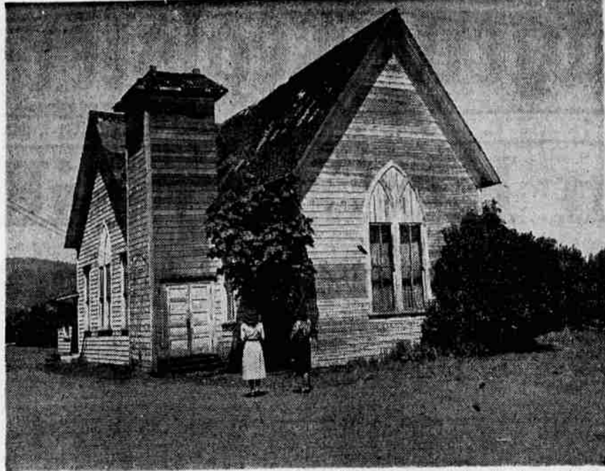
THE OLD CHRISTIAN CHURCH at Thurston, built in 1892, is now being torn down by members of the congregation who will replace it with a modern pumice block church. Taking a last look at the frame building, which was constructed with square nails, is the Register-Guard church editor and the country news editor. Razing started last Saturday and will continue again this weekend. (Staff photo, Wiltshire engraving.)
