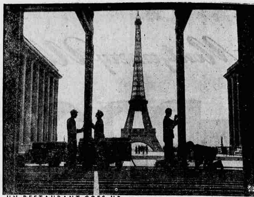
UN RESTAURANT GOES UP —Skeletal structure for a restaurant for the United Nations general assembly delegates frames the Eiffel Tower in Paris. Paris of Palais de Chaillot, which will house the UN sessions are at the left and right.
