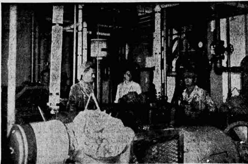
THROUGH THESE PIPES the alcohol-from-wood plant in Springfield passes the 190-proof industrial ethyl alcohol of such vital interest to the nation in time of emergency. The new owner, as yet unknown, will be required to keep the war reserve plant in readiness for industrial alcohol production with 120 days notice by the government. A. E. Buehl, in white shirt, above, operating engineer for the War Assets Administration, supervises a crew of men in preparing the industry for the new owner. Staff photo, Whitlshire engraving.
