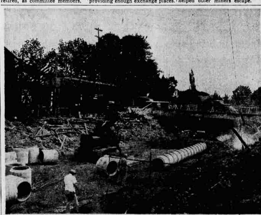
CARS AND TRUCKS will travel above this part of the millrace when the Highway 99 relocation project is completed by the Del R. Beebe Construction Co. This photo shows the pipeline laying operation which will transform the millrace into an underground stream from East Broadway north to Sixth Ave. East of this section of the new four-lane highway, the millrace will again flow in an open channel as it did before its intake canal was ruined in a 1945 Willamette River flood. The culvert being laid here will carry the water on toward the point where it will once again empty back into the river. (Staff photo, Wiltshire engraving).
