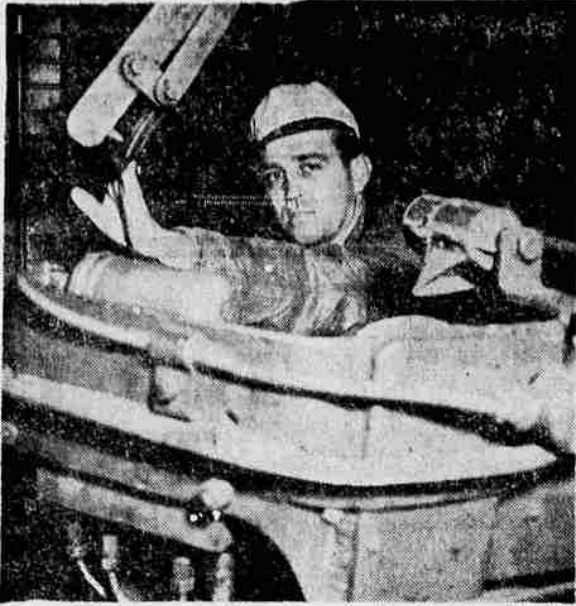
ENGINEER DICK BARNES shoves the throttle forward in the cab of the old burner hauling 74 cars "over the hill." (Staff photos, Wiltshire Engravings.)
