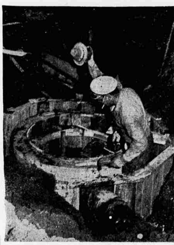
PREPARING FOR AN INFLUX of engineers and dam builders next summer, two workers are putting the finishing touches on the concrete form for a sewer manhole at Lowell. The sewers and other utilities are being installed for the Corps of Engineers housing area by Werner and Jeske of Eugene on a $118,000 contract. (Staff photo, Wiltshire engraving.)
