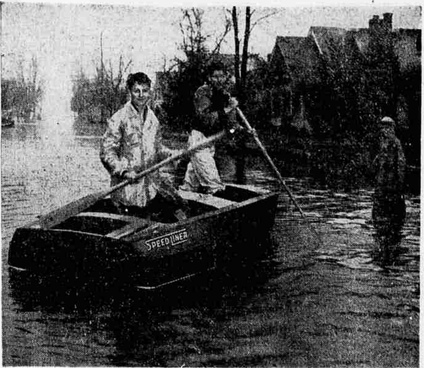
WITH SCHOOLS adjourned, these youngsters enjoyed the flood from their speedboat reconnoitering along south Oak St. where the Amazon Creek spilled over its banks to flood dozens of basements and add to general flood damage.
