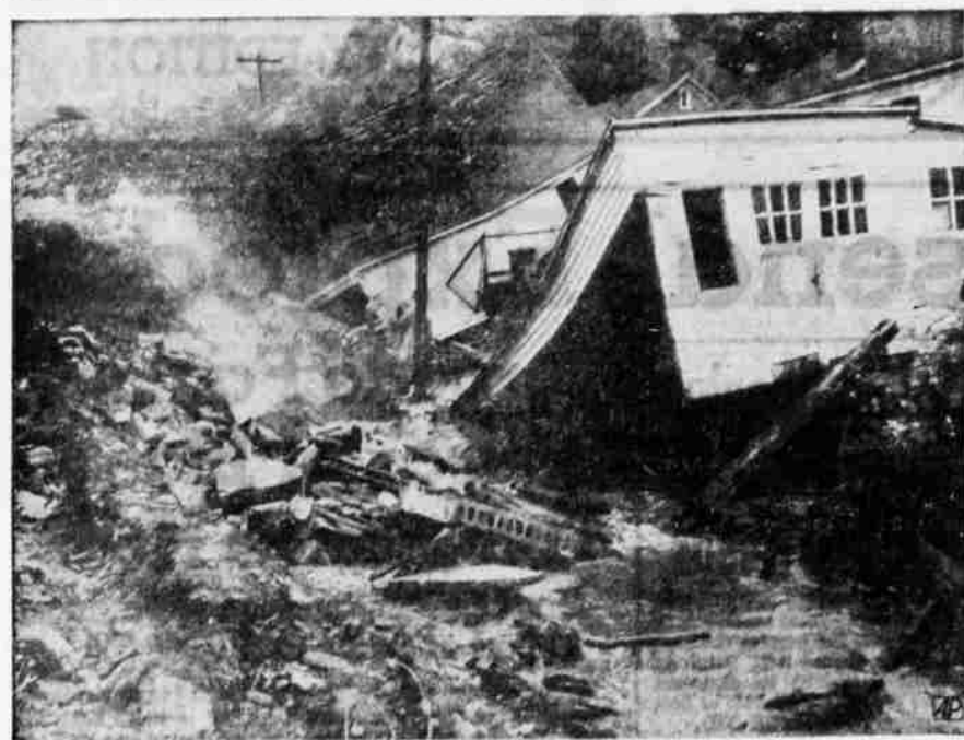
BUILDINGS DIP easily into a gully created by rushing flood water in West Nanticoke, near Wilkes-Barre, Pa., as severe thunderstorms poured four and one-half inches of rain into the Wyoming valley. (AP Wirephoto).
