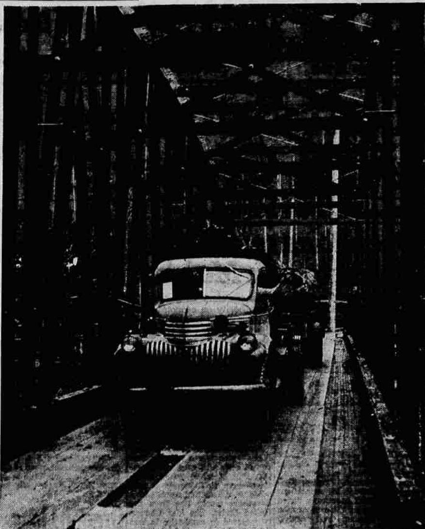
OVER A NEW-TYPE bridge spanning the McKenzie roll logging trucks which were formerly delayed when older bridges gave way during high water periods. The new span features ring connectors instead of bolts and has no piers underneath. (Staff photo, Wiltshire engraving.)
