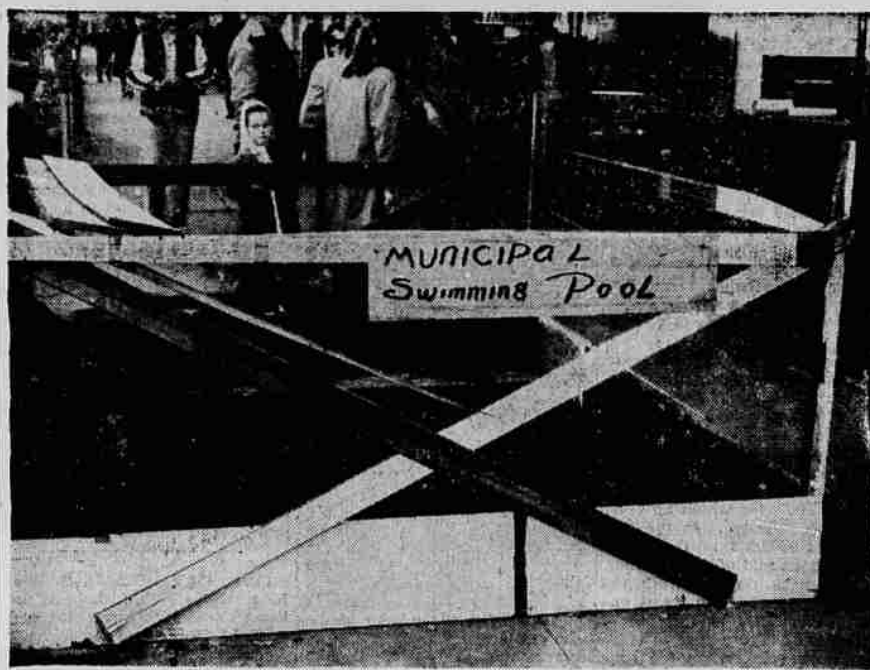
SOME BITTER SOUL just couldn't wait for construction of Eugene's municipal swimming pool, and this excavation at 885 Willamette St. proved too much for him. The sign was attached to the safety fence (to keep out non-swimmers) around the 10 by 10-foot excavation last week. Water in the hole was supplied by plentiful rain. To date, no one has expressed a desire to take the first dip in the new "municipal pool." (Goodwin photo, Wiltshire engraving.)
