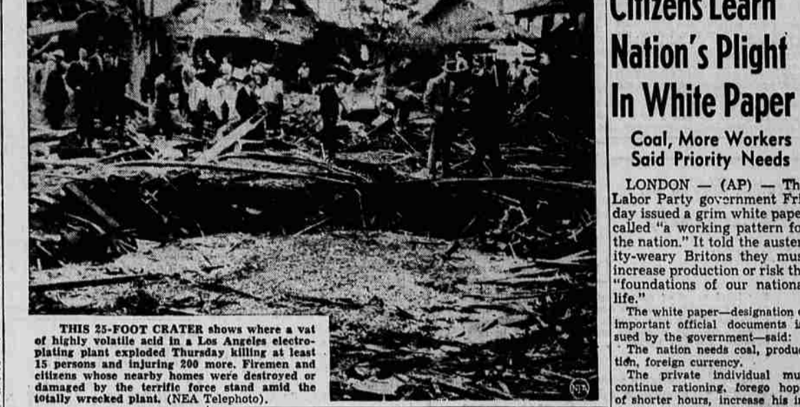
THIS 25-FOOT CRATER shows where a vat of highly volatile acid in a Los Angeles electroplating plant exploded Thursday killing at least 15 persons and injuring 200 more. Firemen and citizens whose nearby homes were destroyed or damaged by the terrific force stand amid the totally wrecked plant. (NEA Telephone photo).
