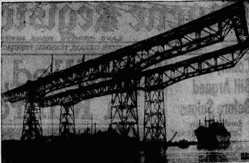
BUILDING GIANT LIFT —The world's largest overhead traveling crane, capable of lifting battleship gun turrets and other huge sections weighing as much as a million pounds, is being erected at the San Francisco naval shipyard, Hunter's Point, Calif.
