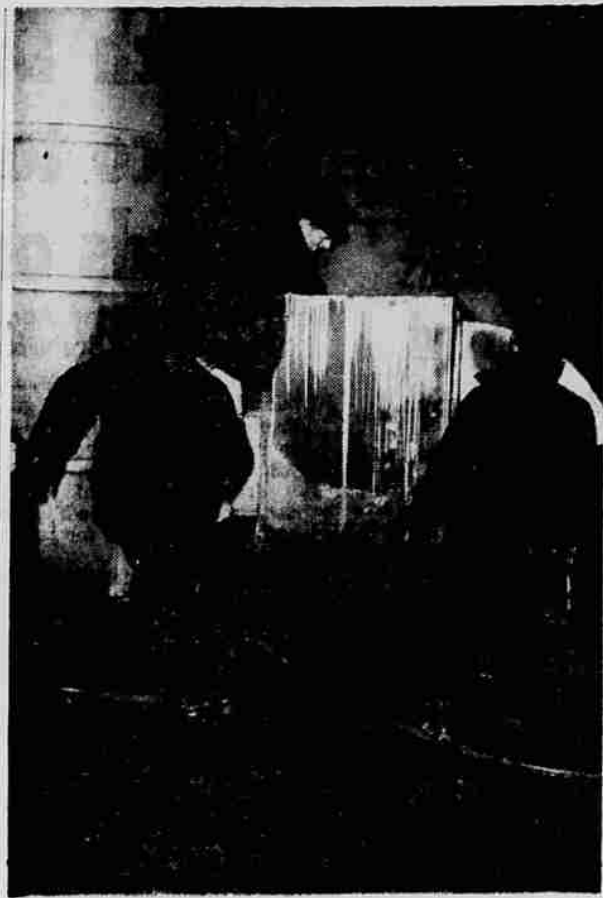
FIREMEN FIGHT ON WILLAMETTE STREET —A main stem blaze which might have been costly was averted at 1041 Willamette St. at 5:24 p.m. Tuesday when city firemen doused a minor roof fire set by as hotted ventilating motor. Incidentally the roof at 1041 Willamette St. covers The Register-Guard.
