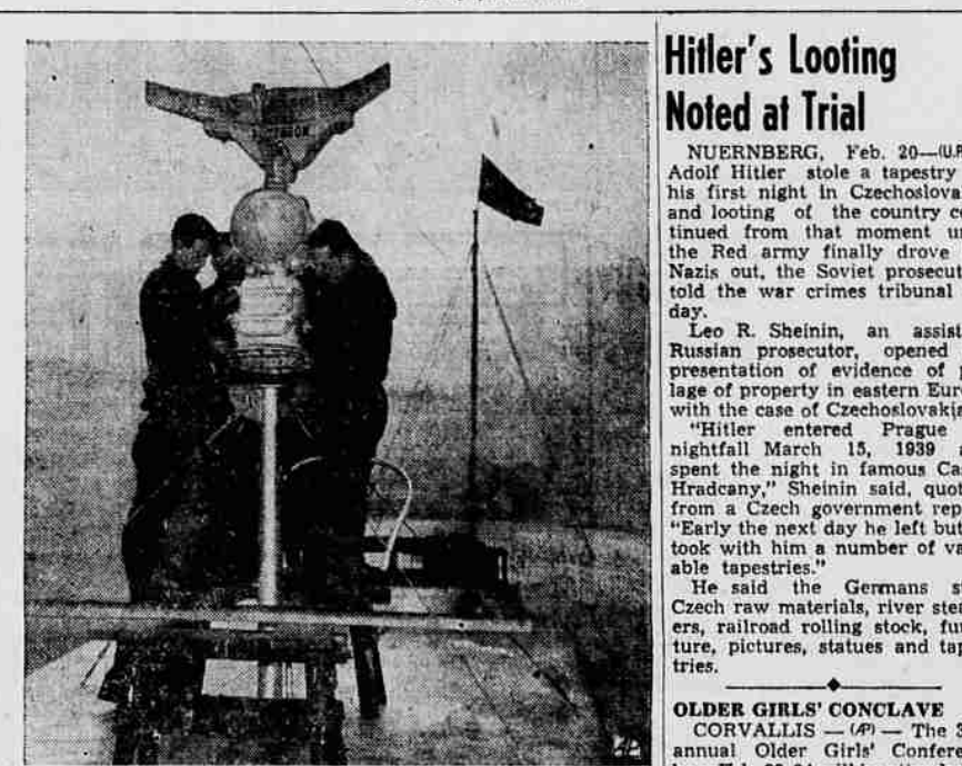
RADAR FOR FERRY —For fog and night operations, technicians of the Black Ball ferry lines of Seattle install radar equipment on the vessel Kalakala in the first peacetime test of the device in Puget Sound.
