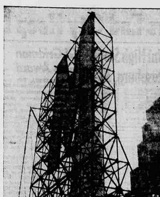
BIG BROADWAY SIGN—Workmen erect the first giant postwar "spectacular" sign on Times Square, New York City, with letters five stories high. The sign will use almost a mile of neon tubing and three miles of cable.
