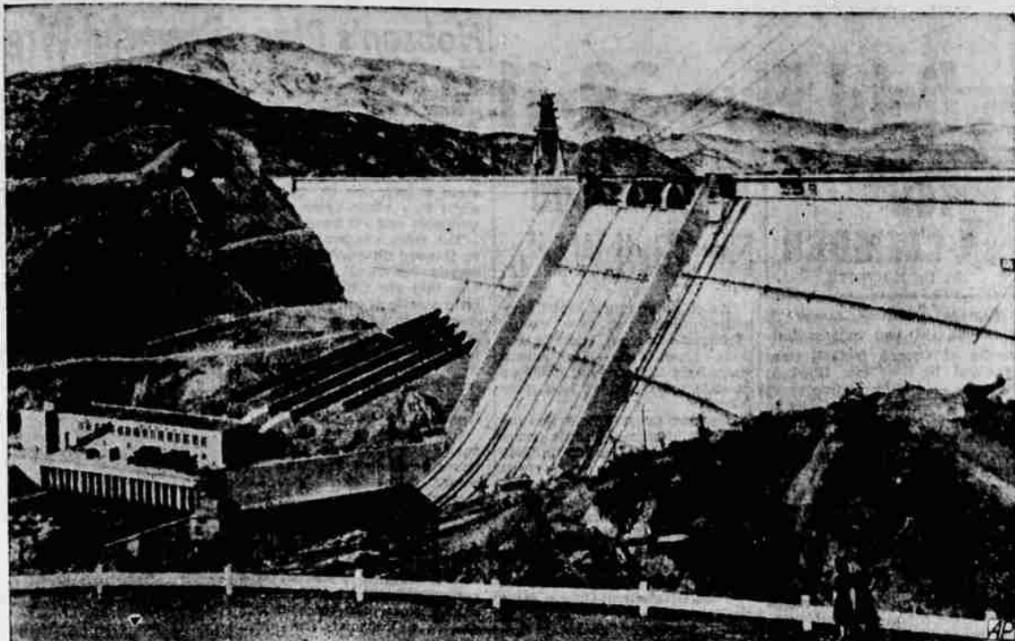
SHASTA POWER FOR WAR PLANTS—This new picture of the Shasta dam in northern California shows it complete except for the three drum gates and the bridge above them. Power plant below furnishes current for San Francisco area war plants.
