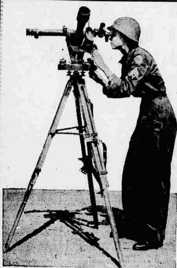
On the antiaircraft firing range, a Wac technician operates a BC Scope, which "tracks" the tow target planes and records hits and misses of Antiaircraft Artillery soldiers.
