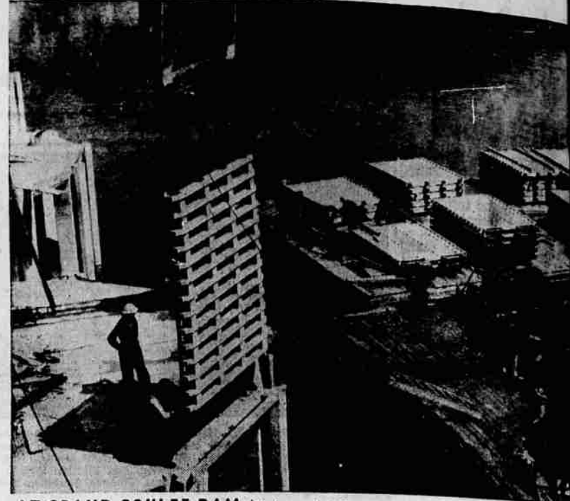
AT GRAND COULEE DAM —Workmen install a temporary track of timber and concrete at an intake of a Grand Coulee Dam, Wash., powerhouse. Steel will replace it later.
