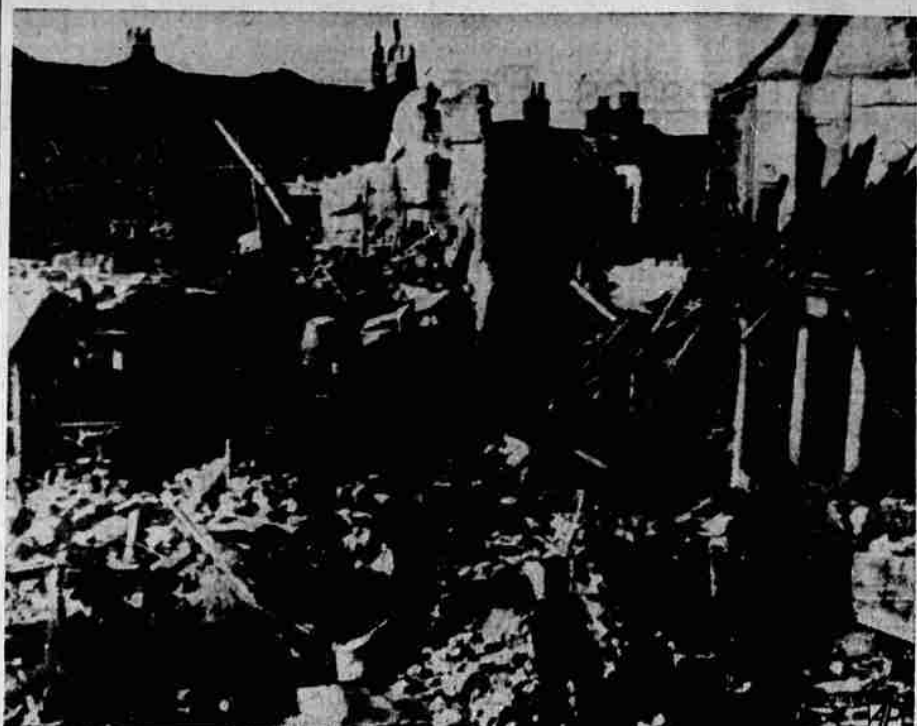
GERMAN BLITZ RETURNS TO LONDON—Workers clear away wreckage of four houses destroyed in one of the heaviest German raids on the British capital in over a year. One woman was killed when these houses were hit. This photo was radioed from London to New York.
