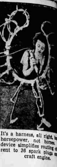
It's a harness, all right, but horsepower, not horse, device simplifies routing of rent to 36 spark plugs on craft engine.
