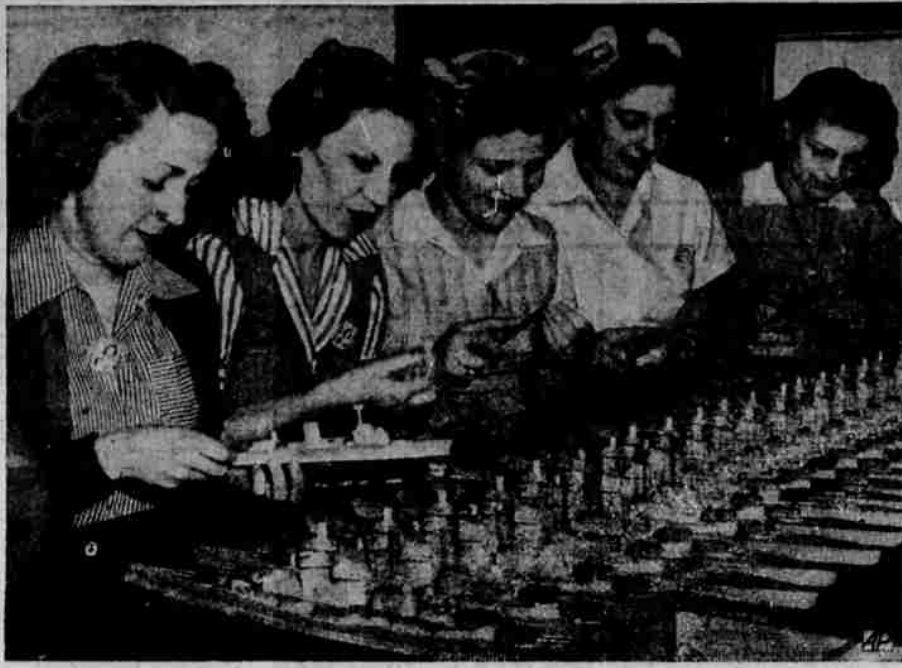
MAKING ENEMY SHIP MODELS FOR NAVY—These women at the Taylor Model Basin at Carderock, Md., make scale models of enemy warships for Navy use.
