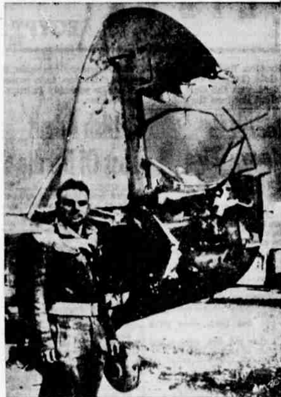
HE MADE A SAFE LANDING —This R. A. F. pilot in Libya brought his damaged Curtis Tomahawk fighter plane down safely although the rudder and elevator were almost shot away, as shown, in action over Sidi Rezech. The plane was damaged by a high explosive shell.
