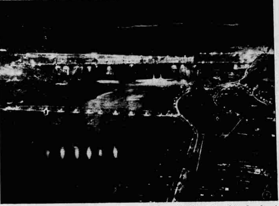
NIGHT FALLS, but work continues under a battery of lights at Grand Coulee dam in Washington, where the mighty structure is rapidly being rushed to completion. By the end of this year the first power will be available from two 10,000-kilowatt house units.
