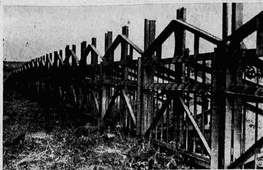
BELGIANS have constructed such steel fences as this along the German border, just in case that nation might forget its pledges to its neutrality.
