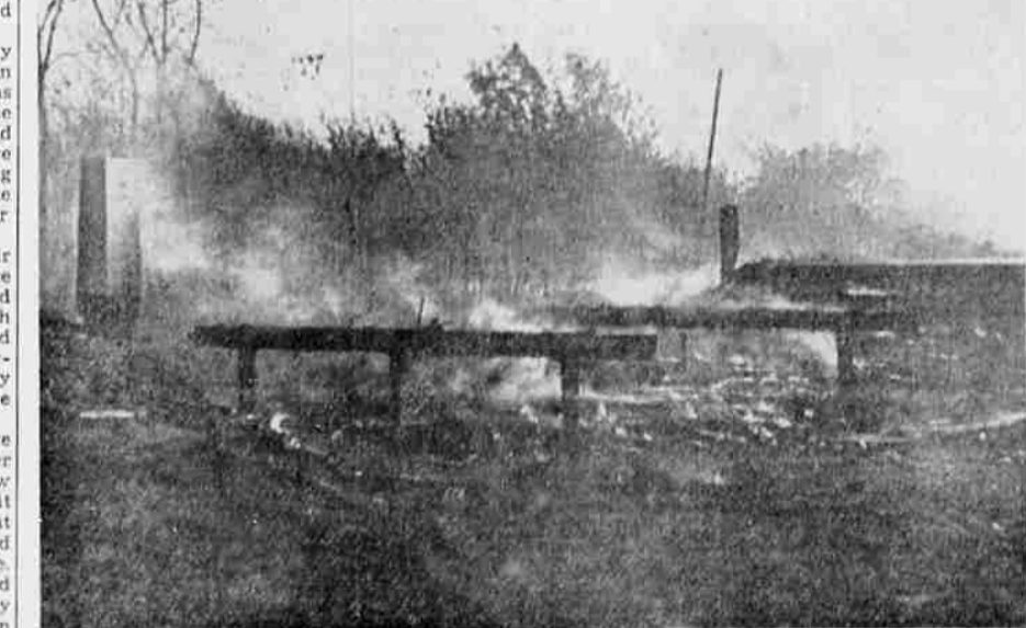
THE area between Eugene and Elmira was ravaged by a serious brush fire Saturday. Here is all which remains of one of two county bridges which burned. Flames covered 2,000 acres. (Photograph by Herbert Wiltshire, Wiltshire engraving)
