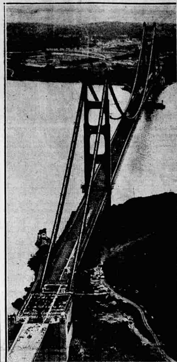
HERE is the latest view of the world's greatest single suspension bridge, built across the Golden Gate at San Francisco at a cost of $35,000,000. Rapidly nearing completion, the bridge will be opened May 1 to traffic. This view was taken above Marion County hills and looks toward San Francisco.
