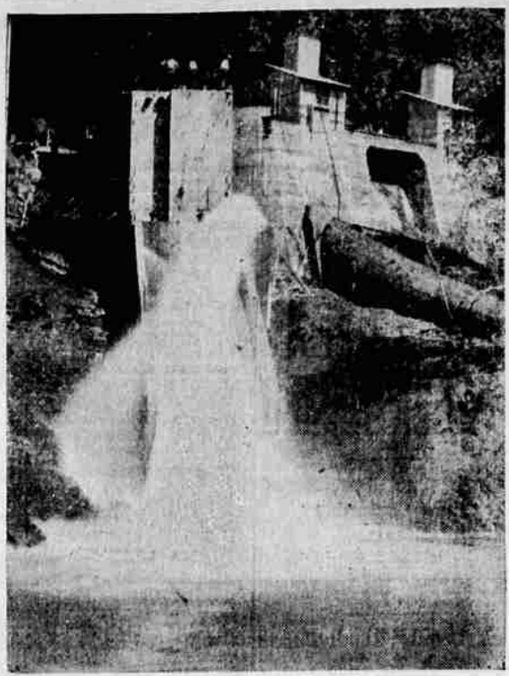
Wiltshire engraving. THE new concrete syphons at the Waltherville power plant are shown here as the water was turned through them recently. The new syphons represent the most modern ideas in spillways and replace the old wood affairs which had served
