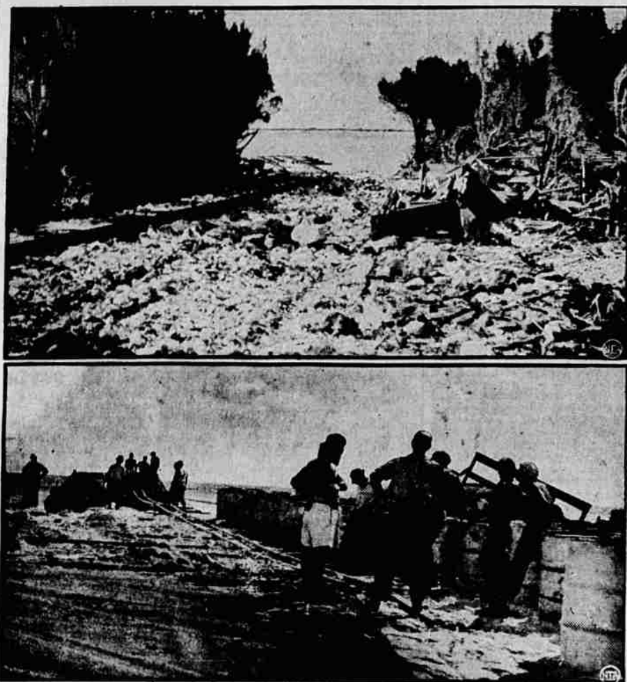
First pictures to reach the Pacific Coast show construction scenes at two of Pan American Airways' airline bases in mid-Pacific Ocean, being established for inauguration of a commercial airway that will soon link the United States and the Orient. Above, clearing a path through ironwood brush on desolate Wilkes Island in the Wake group for a supply railway. Below, unloading thousands of gallons of gasoline at Midway Island awaiting arrival of the first flying Clipper.
