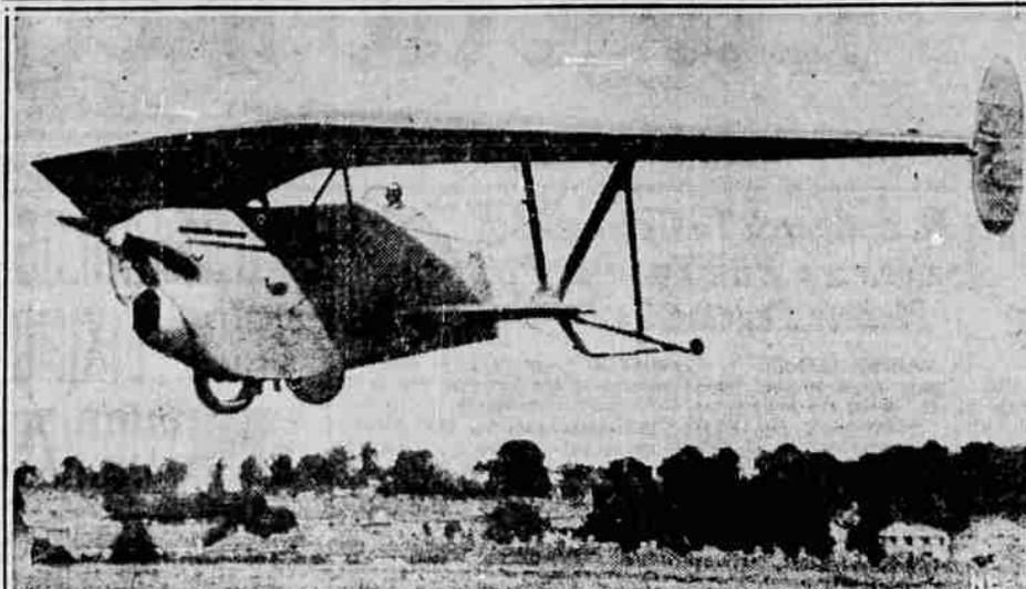
More speed and greater efficiency in the air is predicted by designers for the "pterodactyl" plane, which eliminates the cumbersome fuselage, tail and rudder of the conventional type of aircraft. One of the odd craft is shown in a test flight at Yeovil, England. It is named for the most primitive flying animal known to science.
