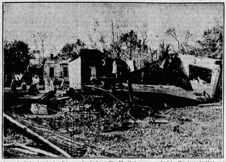
Several of the hundreds of homes in Jacksonville, Ill., that were wrecked by the tornado that swept the vicinity. Although property damage amounted to an estimated million dollars, only eight persons are known to have been seriously injured and no deaths are reported.
