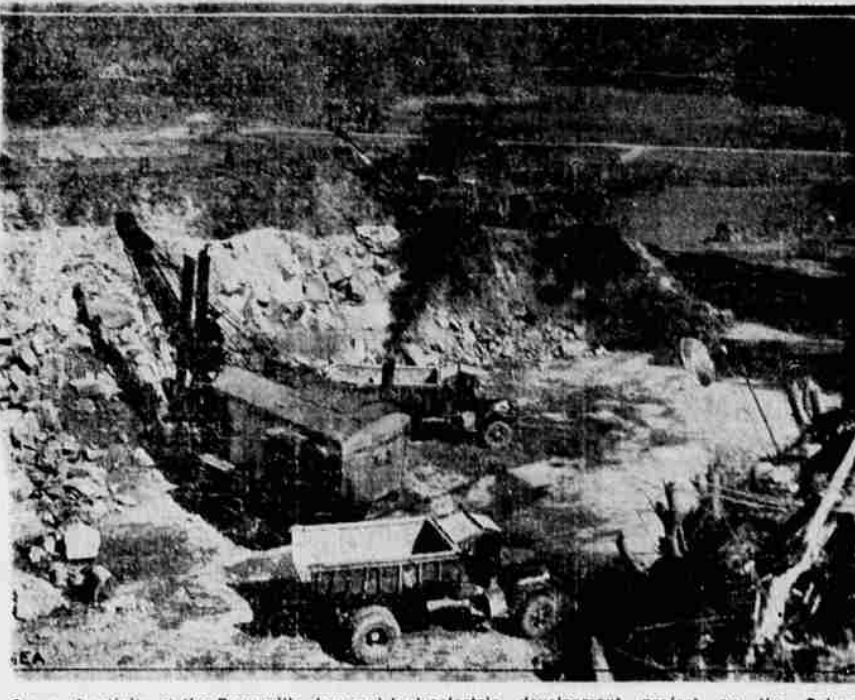
Scene of activity at the Bonneville dam and hydroelectric development project on the Columbia river, Oregon, where 1300 men are engaged in preliminary work harnessing the river. When completed the dam will raise the water level of the river 62 feet, generate 105,000 horsepower and extend slack water navigation range some 100 miles above Portland, metropolis of the district.
