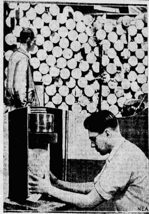
Stringent tests as to shrinkage, tensile strength, reaction to stress and strain, etc., is given the cement under consideration for use in Boulder Dam construction.
