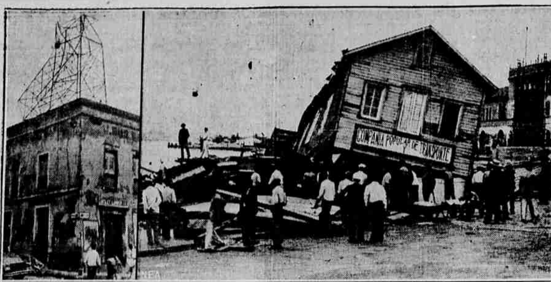
These pictures, rushed by airplane from Puerto Rico, give an idea of the havoc wrought by the hurricane that ripped through San Juan, inflicting millions of dollars worth of damage, killing more than 200 persons and injuring 1000 others.
