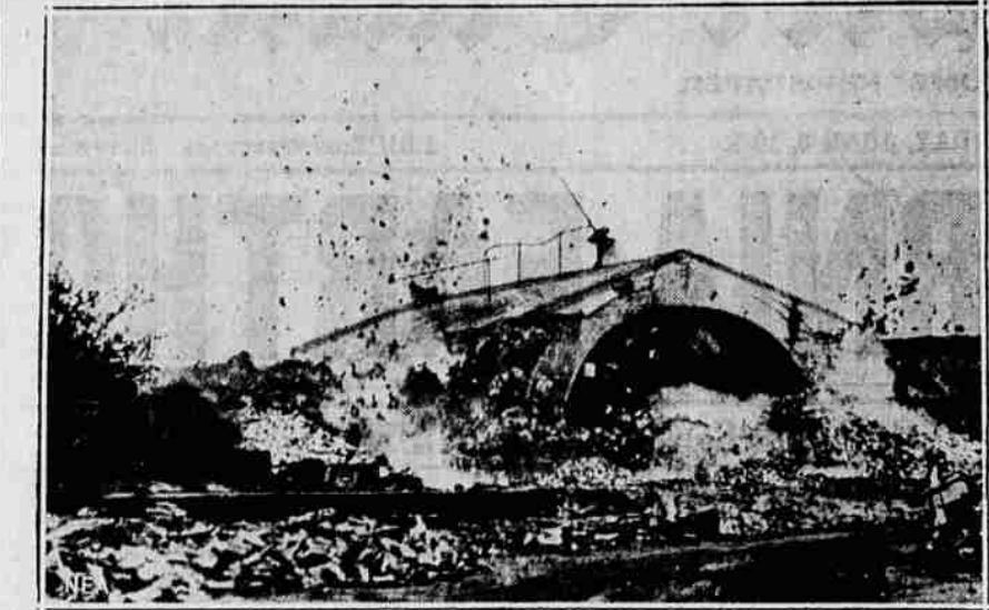
Not enemy shells, but workmen's dynamite was destroying Fort St. Anne at Antwerp, Belgium, when this spectacular picture was snapped. It was part of the Belgian government's program of dismantling fortresses which were erected as defenses during the World War.
