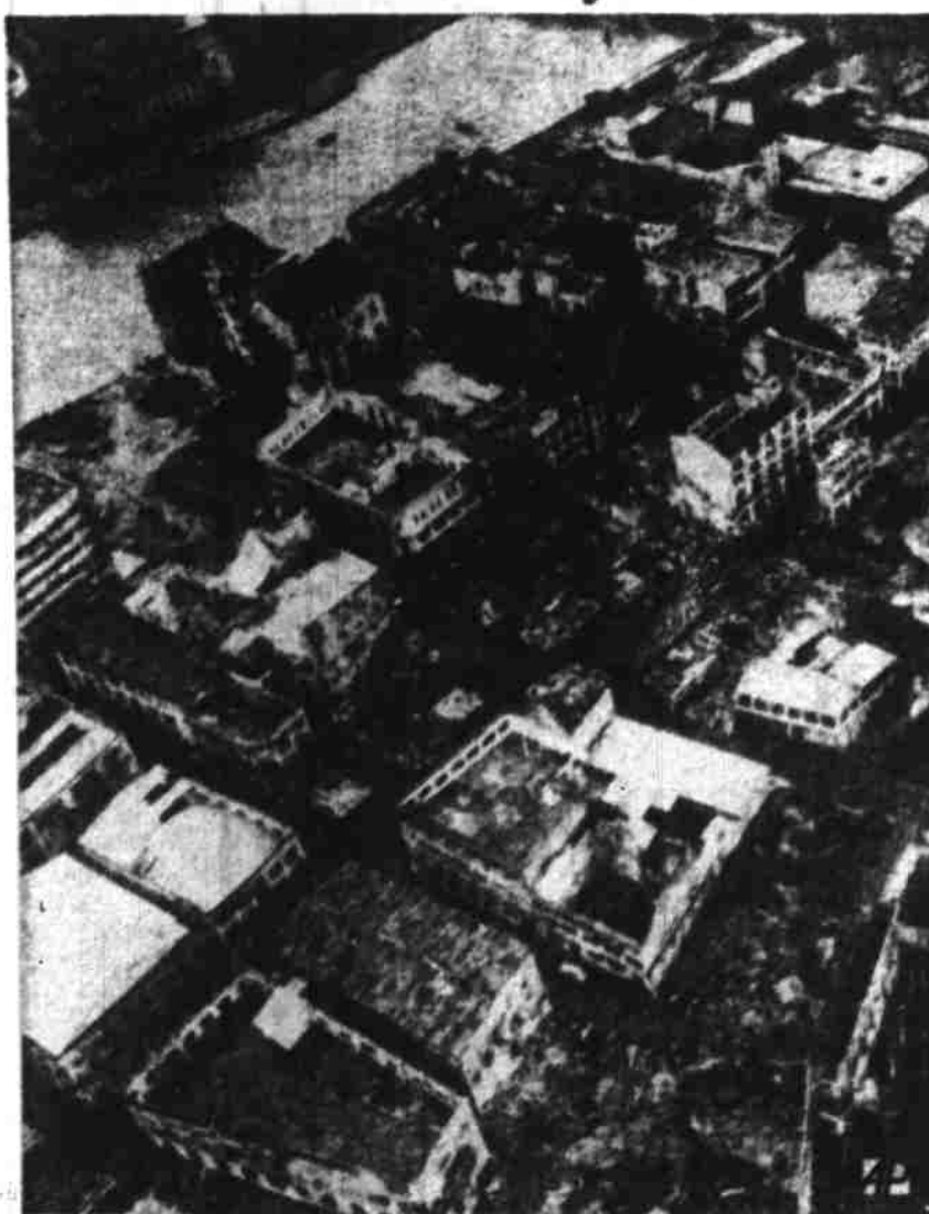
Debris of war still is prominent in downtown Manila on Feb. 1 even as reconstruction work proceeds. Upper left is post office building and directly across the Pasig river is the Philippine National Bank building (scaffolding up), and in left, center, another building leans on its sides. American troops entered Manila on "the road back" on Feb. 3, 1945. (AP Wirephoto)
