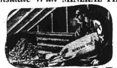
You're paying for INSULATION . . you may as well have it! Mineral fill is easy to install (just pour it from the sack); it's clean, odorless and freproof. Will not disintegrate or support vermin. Bag covers 18 sq. ft., 3" deep.
