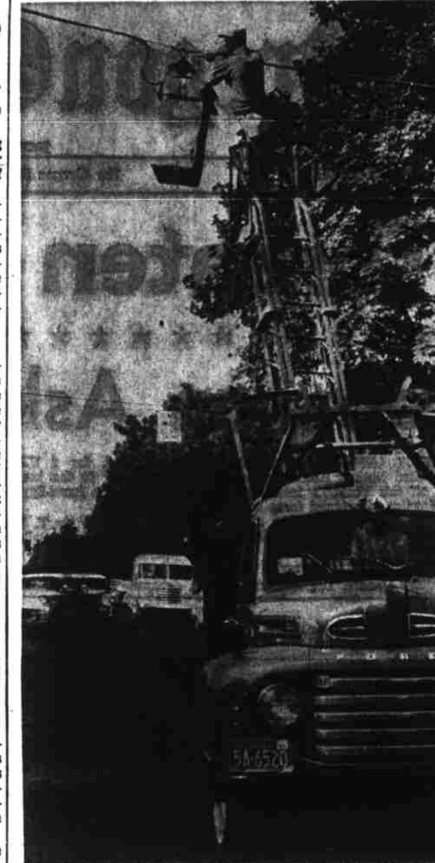
Workmen unmask new traffic lights at the intersection of Cottage and State streets before putting them in service late Wednesday. Earlier in the day, new lights at Court and Cottage streets were put in working order. (Statesman Photo)
