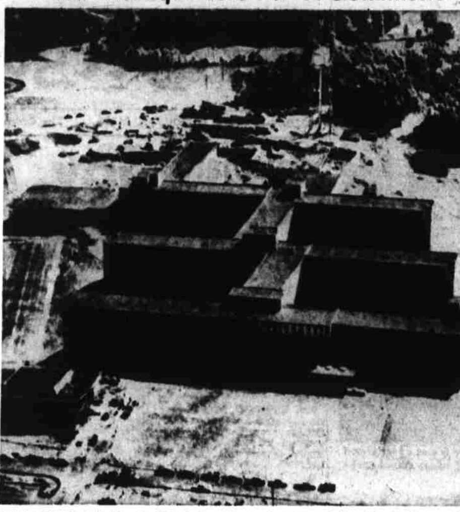
GERMANTOWN, Md., Nov. 5—This is the new headquarters of the Atomic Energy Commission which President Eisenhower will dedicate on Nov. 8. The $13,300,000 structure near Germantown, Md., is of reinforced concrete, faced with brick. Some 1,500 employees will move into the building in January. (AP Wirephoto)
