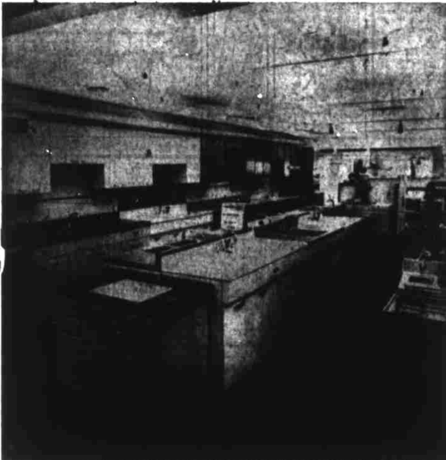
Enlarged and modernized plumbing section in basement of completely remodeled Montgomery Ward store in downtown Salem. The store will celebrate its grand re-opening Wednesday noon.
