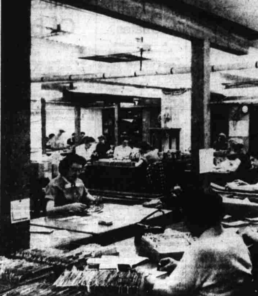
One of the areas of the State Office Building which Secretary of State Mark Hatfield Monday labeled "unhealthy" because of overcrowding and poor ventilation was this basement office occupied by state tax workers. Wooden pillars shown were placed in the basement last year when the ceiling began to crack. (Statesman Photo)
