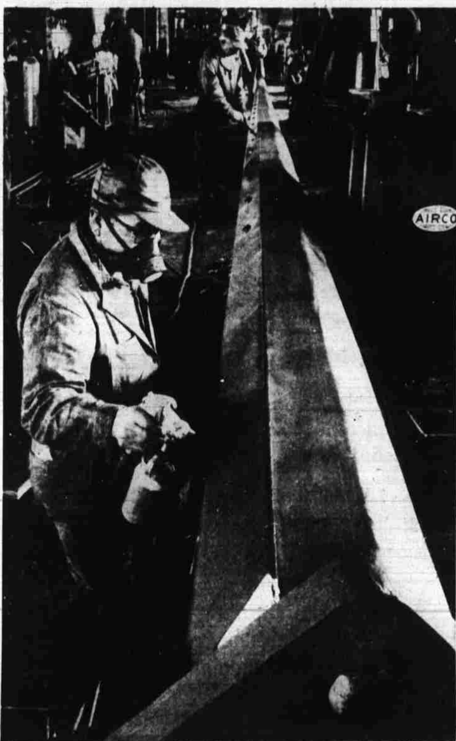
Probably one of the largest poles of its kind ever constructed in the Northwest, this giant 80-foot steel electric pole is one of six now being fabricated at Hrubetz & Bushnell Manufacturing Co., 2380 S. 25th St. Joseph Sanders (foreground) is spraying the monster. (Statesman Photo)
