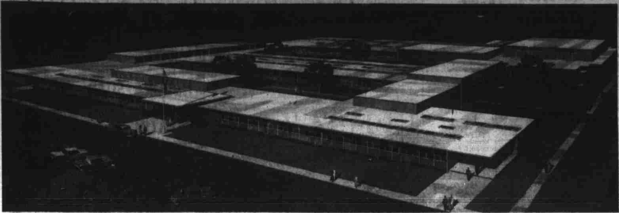
Here's what Salem's two new $1,000,000 junior high school buildings will look like. Bids will be opened on the nearly identical structures Nov. 19 at a special meeting of the Salem School Board and construction is expected to get underway immediately, according to Supt. Charles D. Schmidt. Perspective above is actually of Waldo Junior High which will be located on Lansing Avenue near Wash-
